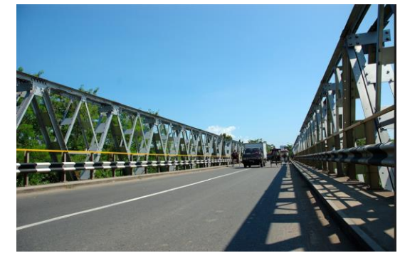
Steel bridges, guard rails
