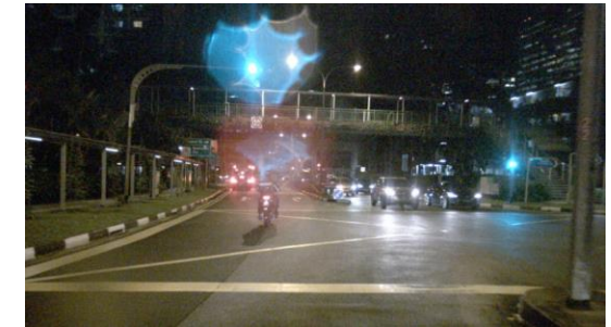
Metal structures + rainy weather + bad lighting conditions
