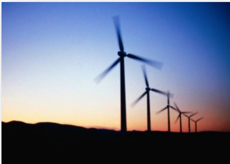
Turbines on a wind farm.
